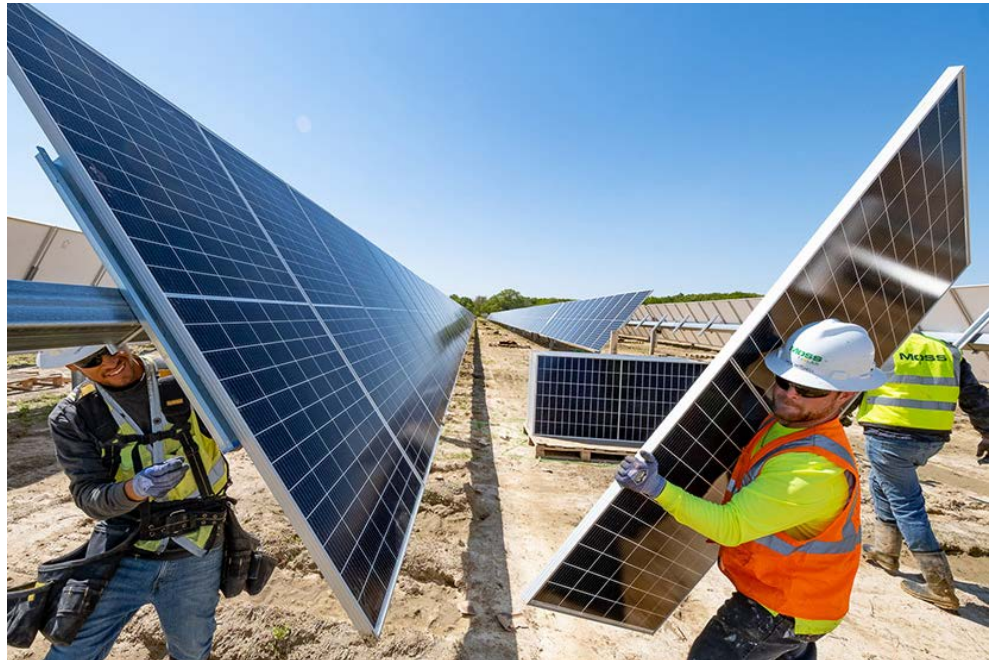
Construction of Entergy Arkansas' Searcy Solar Energy Center | Entergy
