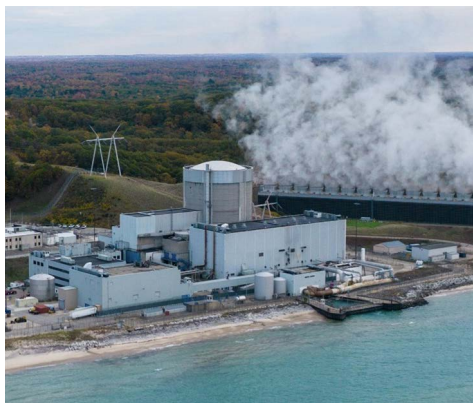
The Palisades nuclear plant in Covert, Mich. | Holtec International
