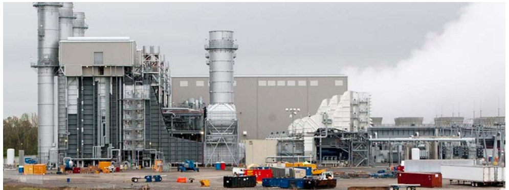
The Paradise Combined Cycle Plant in Drakesboro, Ky. | TVA
