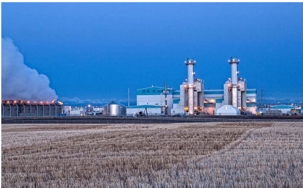
A WECC winter-weather readiness webinar featured a discussion of the Alberta Electric System Operator's response to the severe cold snap of January 2024. AESO is heavily dependent on gas generation during cold weather. | Electricity Canada
