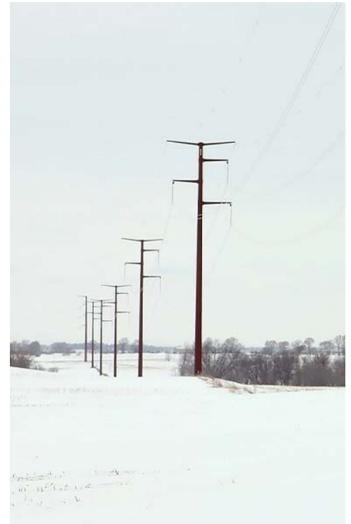
The 345-kV Big Stone South to Ellendale line in the Dakotas | Otter Tail Power Co.
