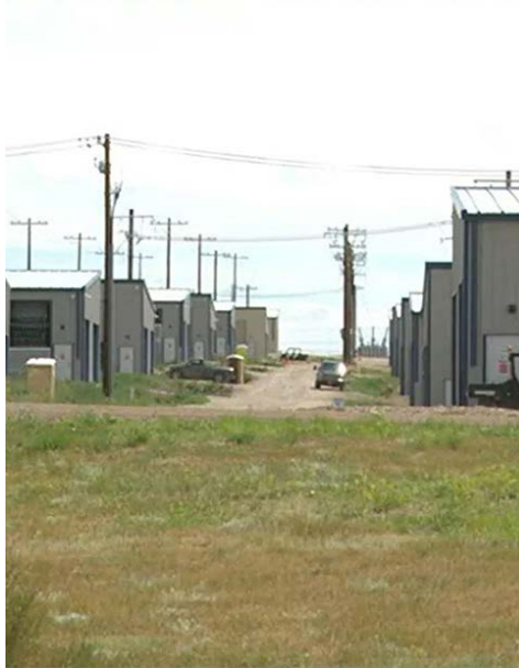
The Atlas Power Data Center in Williston, North Dakota | KFYR TV
