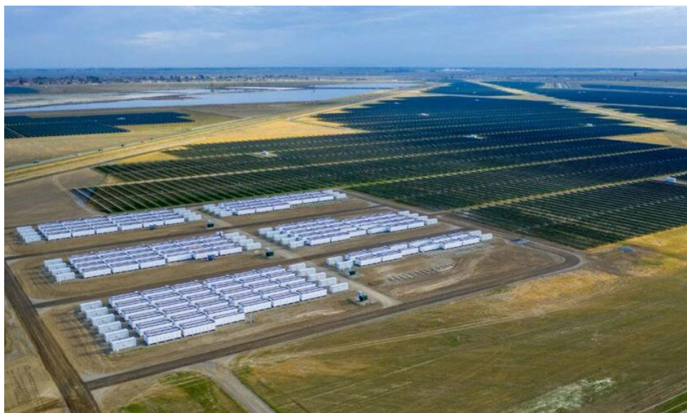
Slate solar-and-storage project in Kings County, Calif. | Goldman-Sachs Renewables
