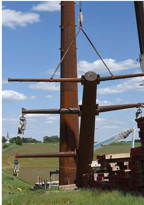
Construction of the Cardinal-Hickory Creek transmission line | ATC and ITC Midwest
