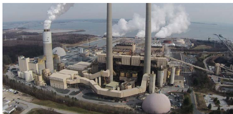
The Brandon Shores coal-fired power plant | Talen Energy
