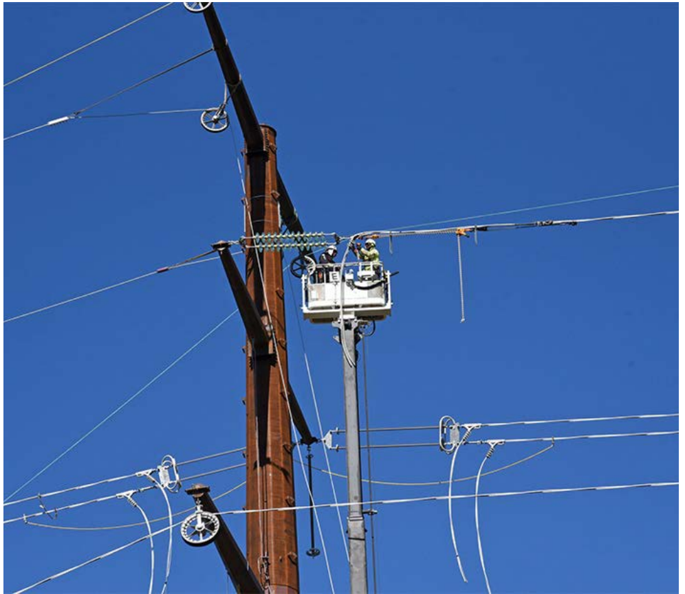
Construction on the Cardinal-Hickory Creek transmission line | American Transmission Co.
