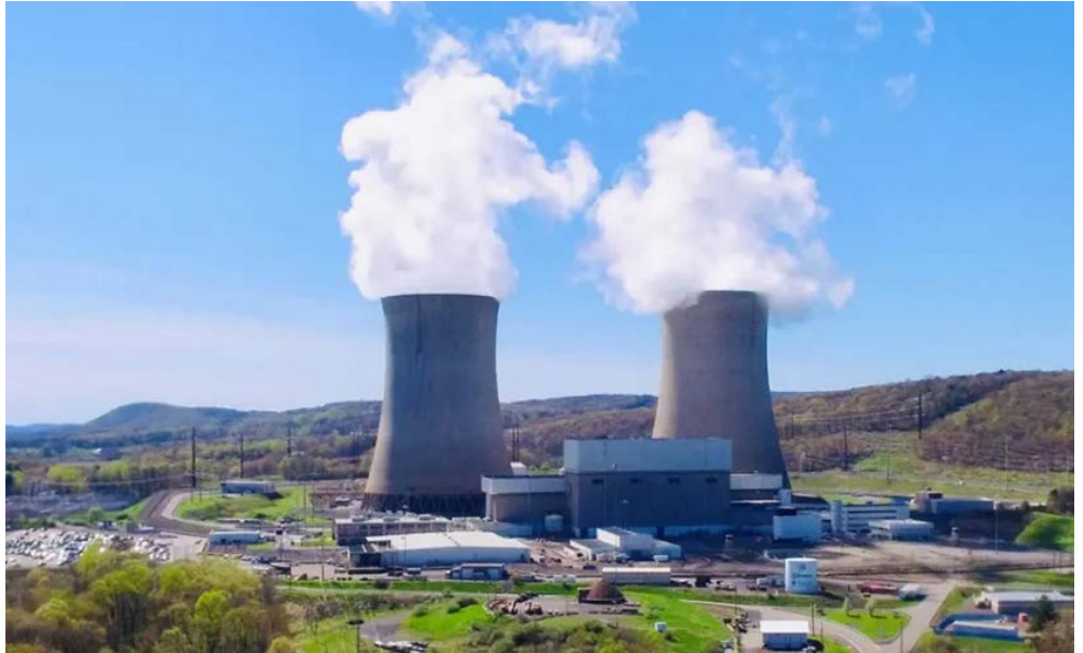
Co-location of data centers with zero-emissions energy resources such as the Susquehanna nuclear power plant was discussed during a WECC webinar. | Talen Energy
