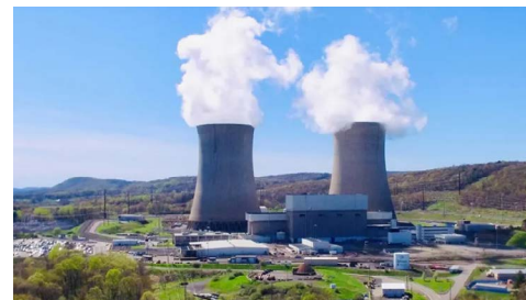
Susquehanna nuclear power station | Talen Energy
