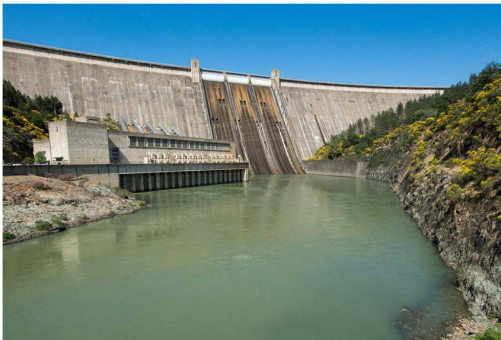
WAPA’s Shasta Dam in Northern California | WAPA
