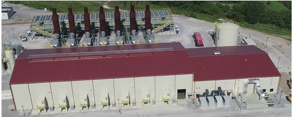
Entergy's New Orleans Power Station under construction around 2020 | Entergy
