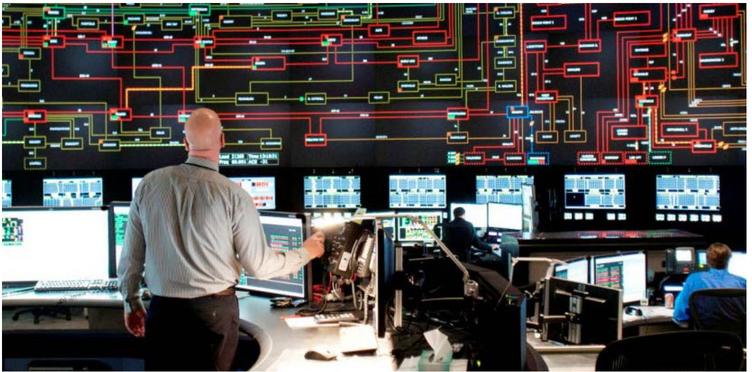
NYISO control room in Rensselaer, N.Y. | NYISO
