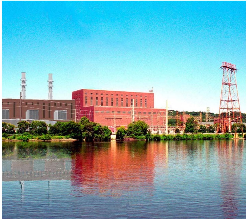
PSEG's Bethlehem Energy Center, an 817-MW combined cycle plant in New York | PSEG
