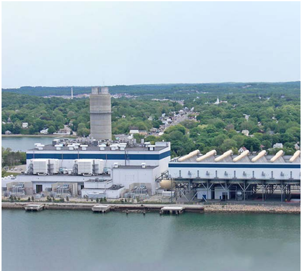
Fore River Energy Center in Weymouth, Mass. | Calpine
