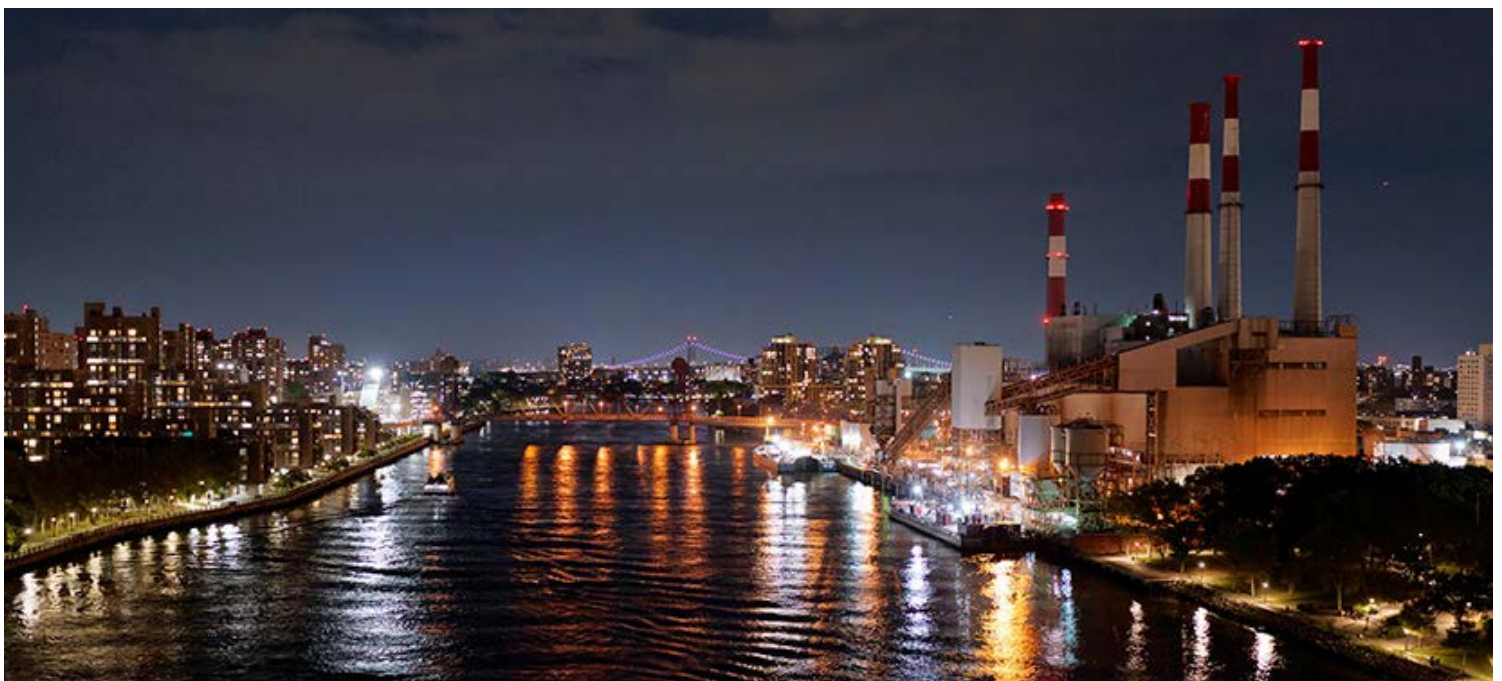
Ravenswood Generating Station in Queens, N.Y. | © RTO Insider LLC
