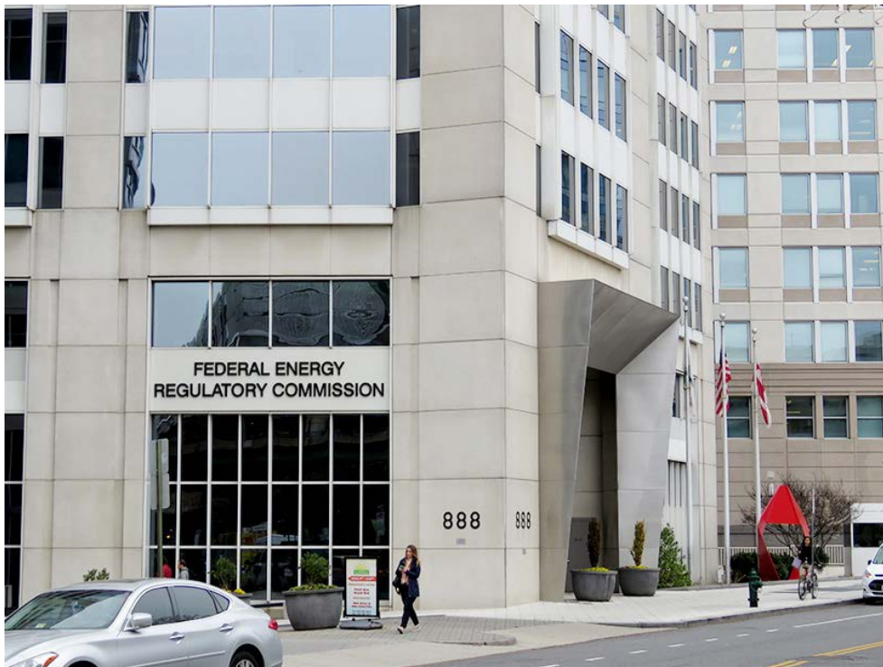
FERC headquarters in D.C. | © RTO Insider LLC
