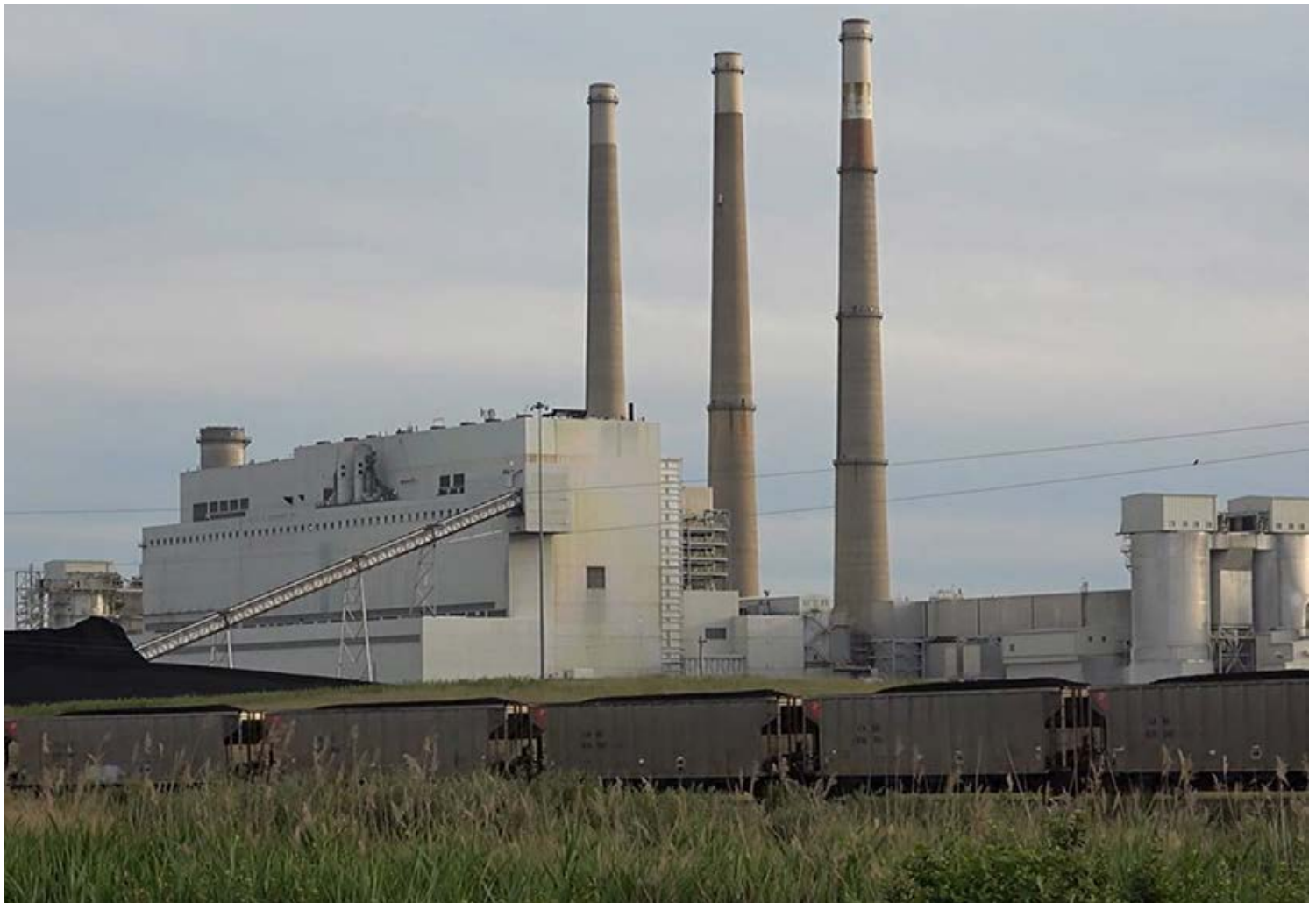
A train passes the Baldwin Power Plant in Illinois. | TrainManBrodie via YouTube
