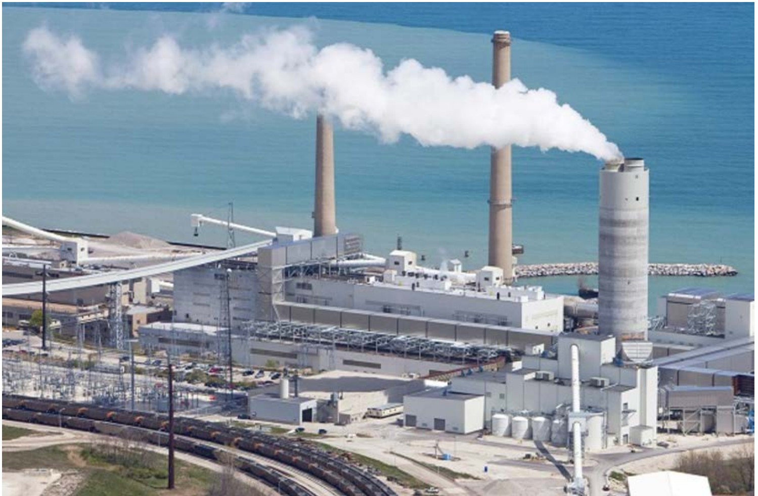
Oak Creek Power Plant | We Energies
