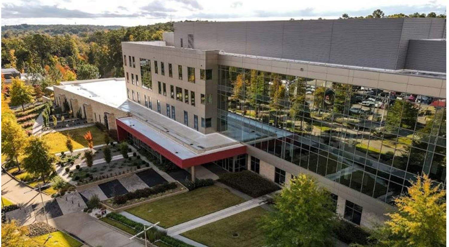
SPP headquarters in Little Rock, Ark. | SPP
