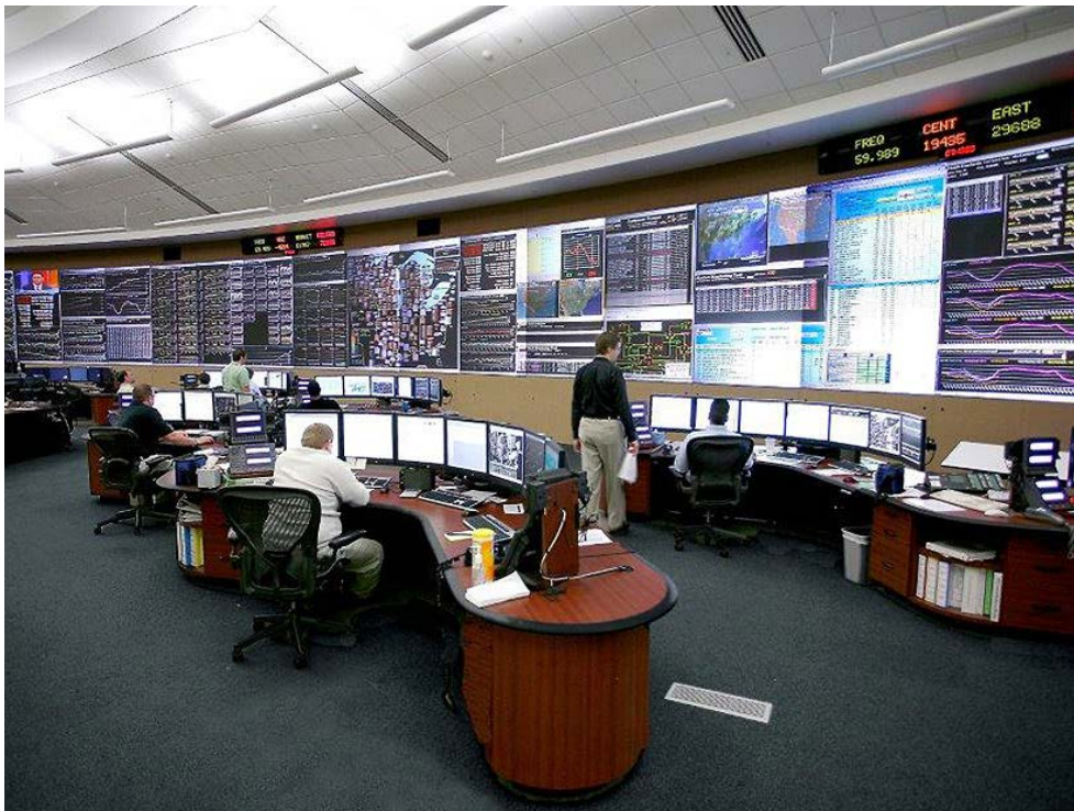
MISO control room | MISO
