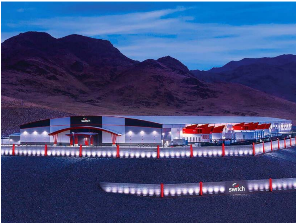
The Citadel data center located in Tahoe Reno, Nev. | Switch
