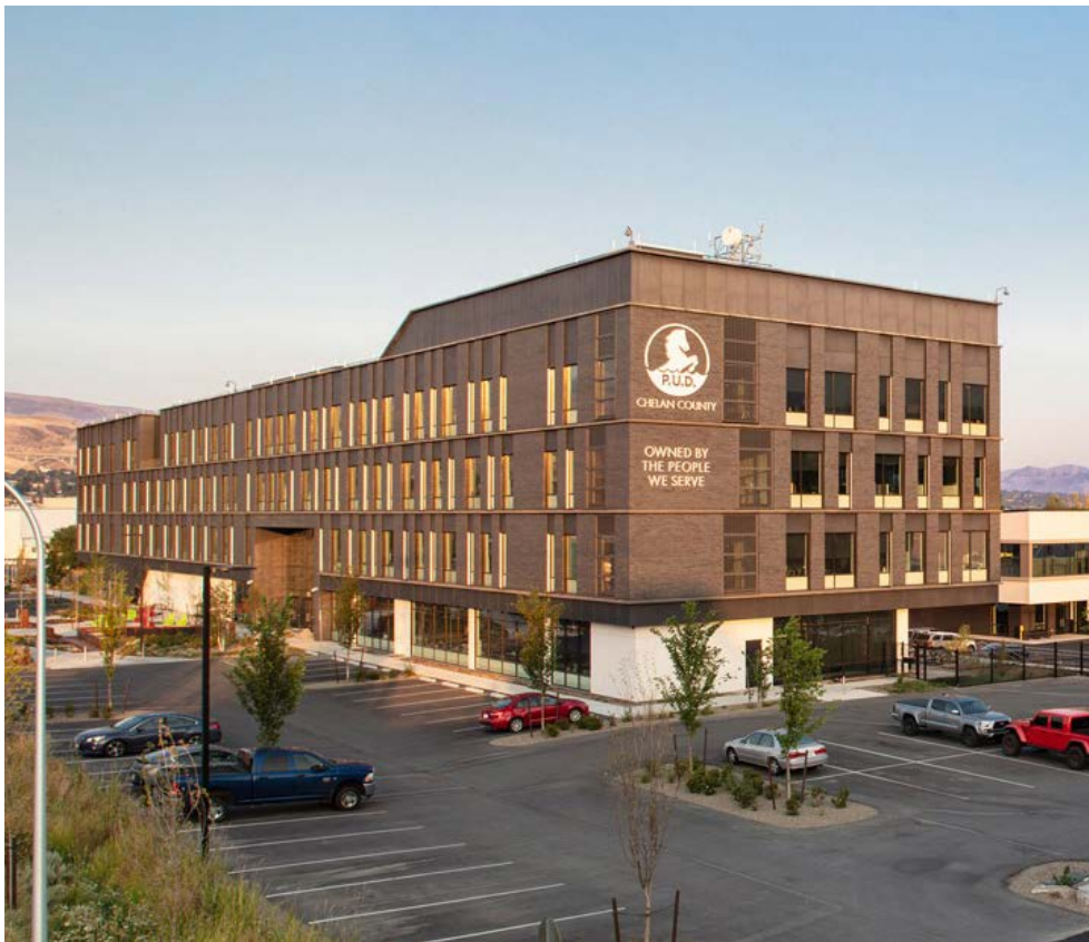
Chelan County PUD's headquarters in Wenatchee, Wash. | TCF Architecture
