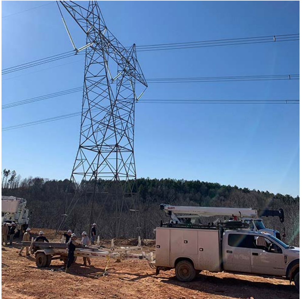
TVA crews rebuilding lines in 2020 after tornadoes in Middle Tennessee | TVA
