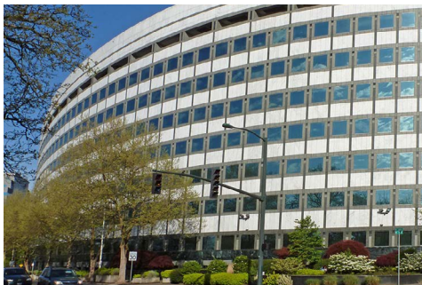
BPA headquarters in Portland, Ore. | Bonneville Power Administration
