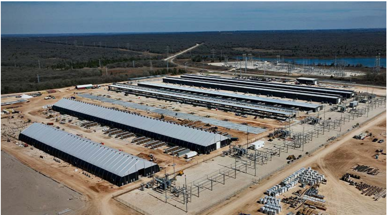
Riot Platform's Rockdale Facility near Austin has a load of 700 MW. | Riot Platform
