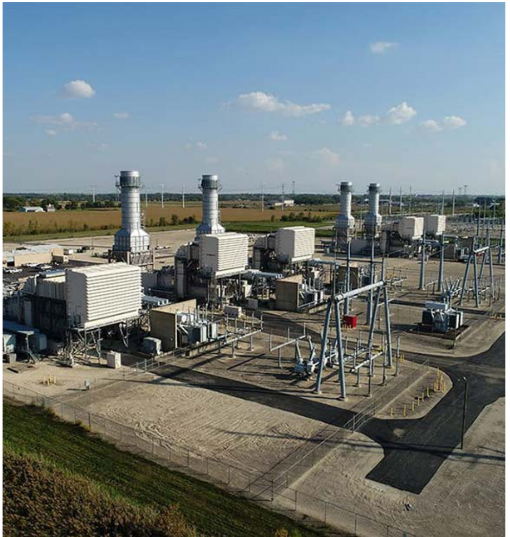
J-Power's Elwood Energy Center, a 1,350-MW natural gas turbine in Illinois | J-Power
