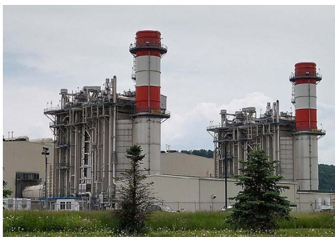
The Panda Patriot Power Plant, a natural gas-fired power station located in Clinton Township, Pa. | Casey Monaghan, CC-BY-SA 2.0, via Wikimedia
