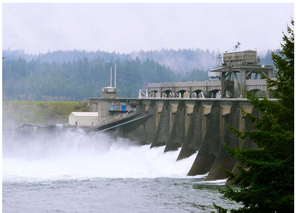
BPA's Bonneville Dam | © RTO Insider LLC
