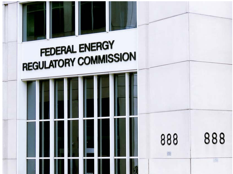
FERC headquarters in D.C. | © RTO Insider LLC
