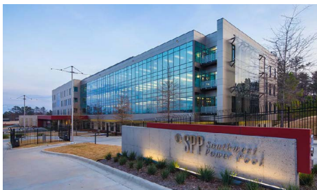
Xcel Energy subsidiary Public Service Company of Colorado (PSCo) has asked the Colorado Public Utilities Commission for permission to join SPP's Markets+. | SPP
