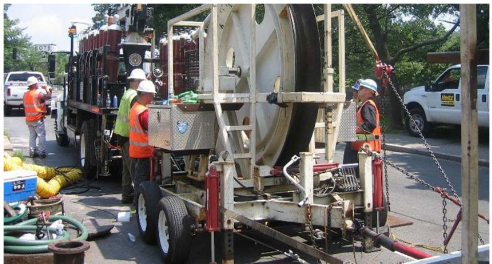
HPFF cable installation | Eversource
