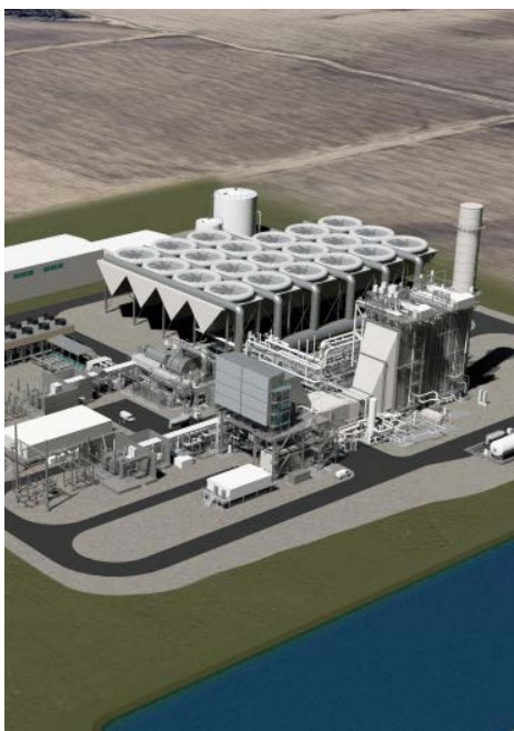
A rendering of Entergy Mississippi's plans for its first power plant in 50 years, the 754-MW, $1.2 billion Delta Blues Advanced Power Station. Entergy has already broken ground for the gas plant. | Entergy Mississippi, Sargent & Lundy
