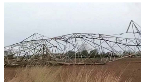
An Entergy Arkansas downed tower on April 3, after severe storms. The extreme weather did not trigger load shed. | Entergy Arkansas
