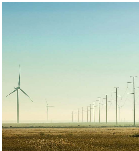
PNM's Western Spirit transmission line. | New Mexico Renewable Energy Transmission Authority
