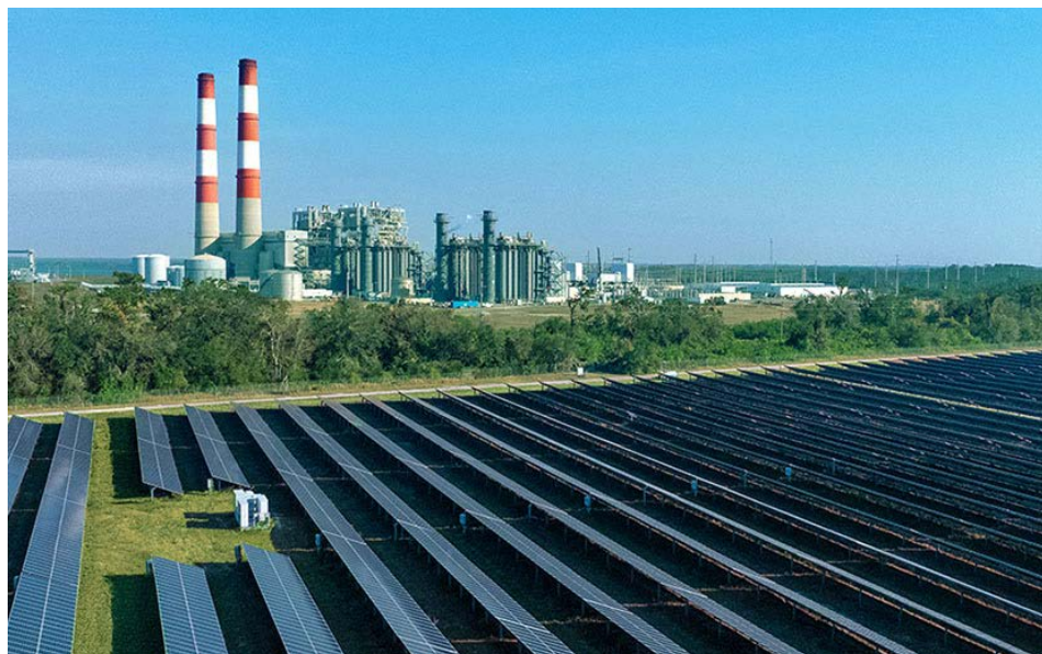
Solar and gas-burning generation facilities owned by Florida Power and Light are shown in Parrish, Fla. | NextEra Energy Resources
