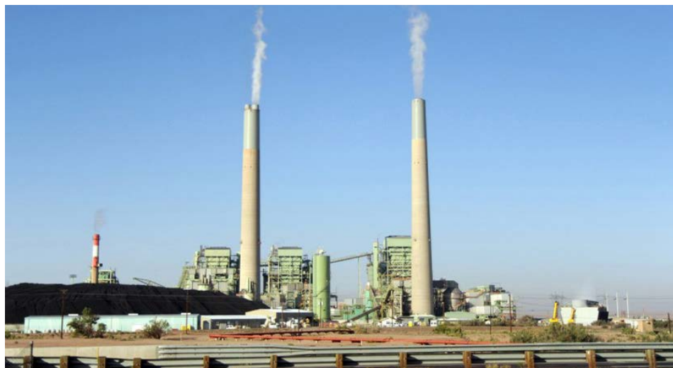
APS' coal-fired Cholla power plant | Center for Land Use Interpretation
