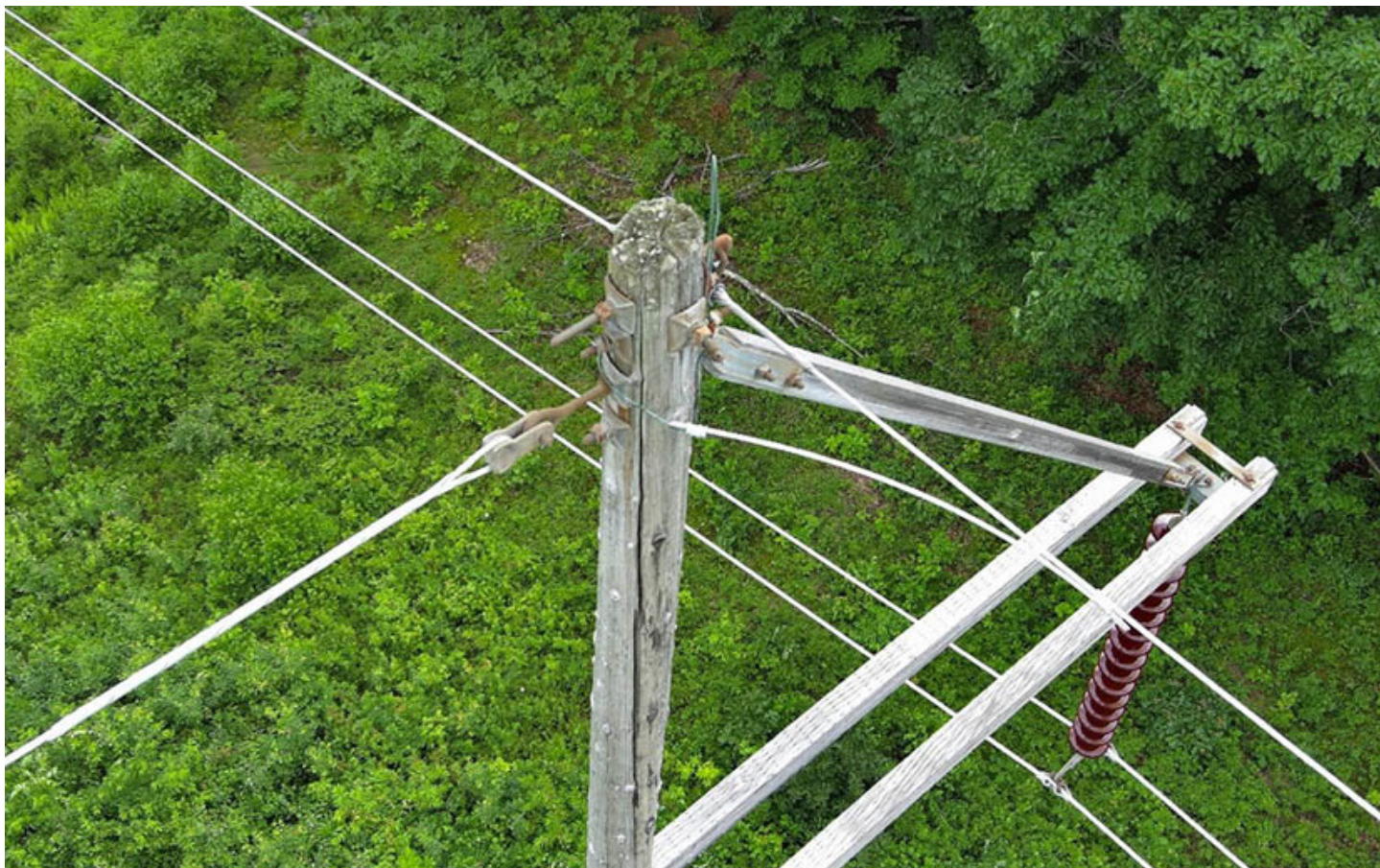
A cracked wooden pole on an Eversource transmission line in New Hampshire | Eversource Energy
