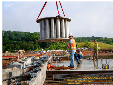
Crews from Kairos Power and Barnard Construction install the reactor vessel support system for its third Engineering Test Unit in May in Oak Ridge, Tenn. | Kairos Power
