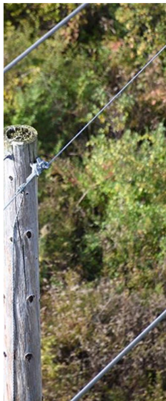
Deteriorating wood structures on a 115 kV line in Rhode Island | Rhode Island Energy
