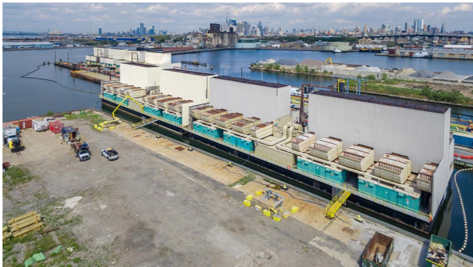
Gowanus barge-mounted natural gas generating station in Brooklyn, N.Y. | Astoria Generating Company
