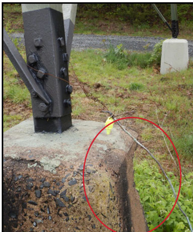
Line 1670/1771 Structure 4133 Foundation Damage
