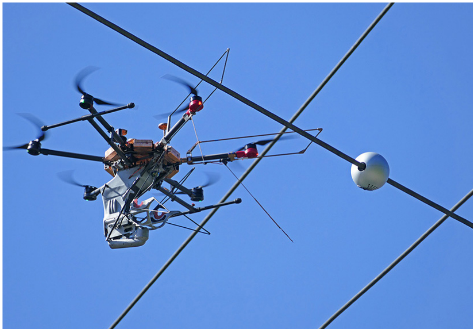
A Heimdall drone installing a monitoring device on a PSE transmission line. | Puget Sound Energy
