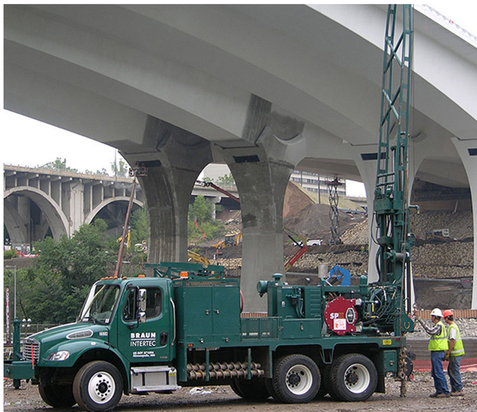
Preconstruction soil boring work | Minnesota Power
