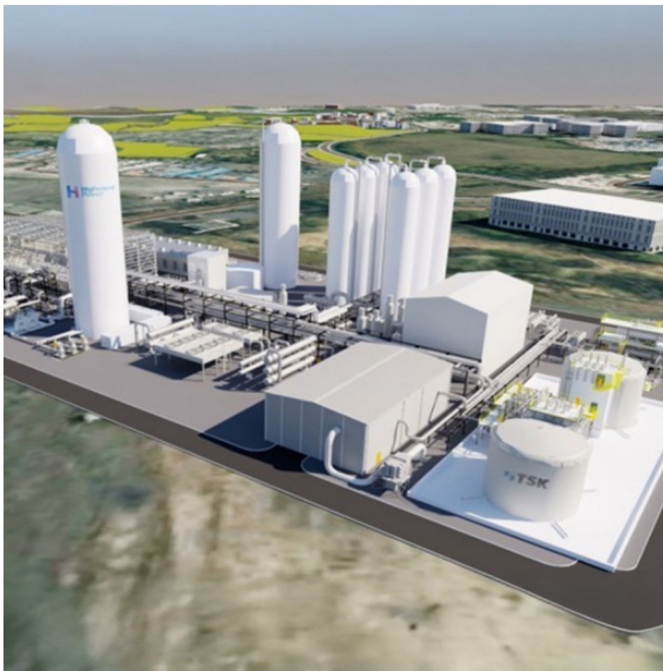
Highview Power is building the first commercial-scale liquid air energy storage plant in the United Kingdom, the 50-MW/300-MWh Carrington project near Manchester. | Highview Power
