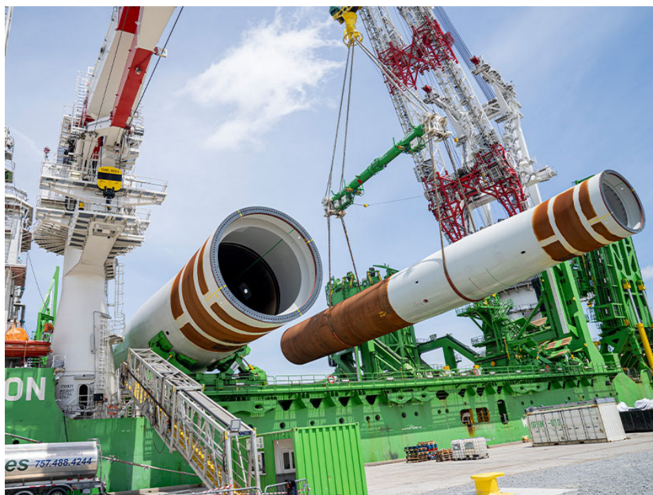
Crews in Portsmouth, Va., load monopile foundations for Dominion's Energy's Coastal Virginia Offshore Wind, which would be the largest wind farm in U.S. waters. | Dominion Energy
