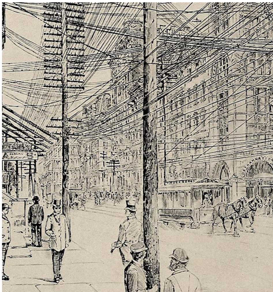
Hundreds of utility lines crisscross a New York City thoroughfare in this circa 1890 drawing. The chaotic tangle of wires serving individual homes and businesses eventually prompted business model and regulatory reforms, leading to the consolidation of competing electric companies into Consolidated Edison in 1936. | Public Domain via Wikimedia Commons
