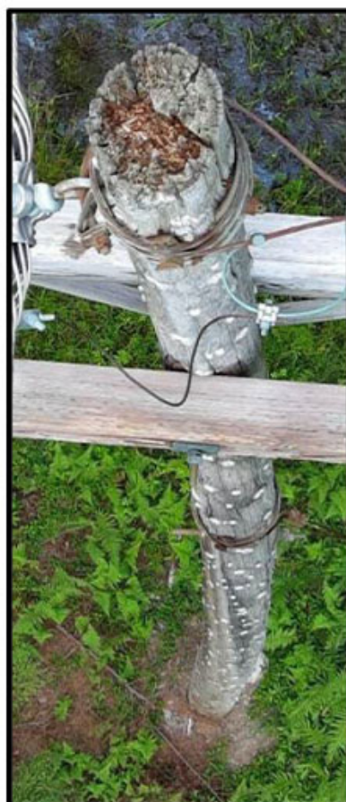
Line B143 Structure 24 Pole top rot and splits, bending
