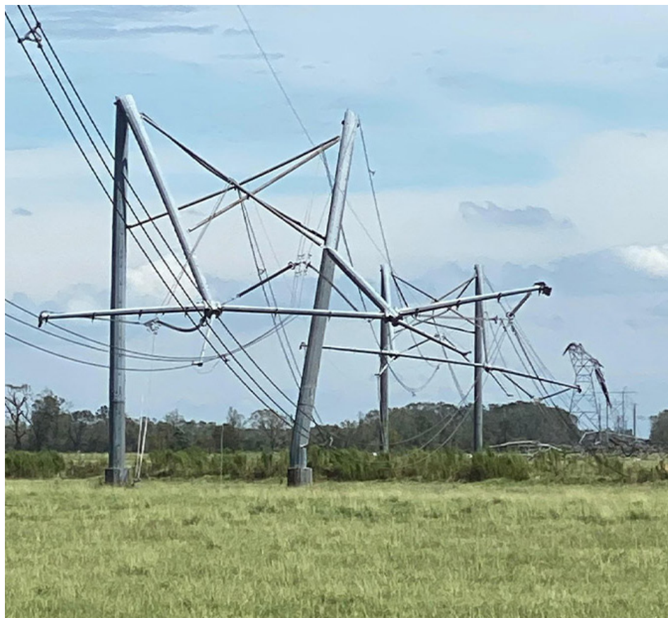
Grid damage in Calcasieu Parish following Hurricane Laura in 2020 | Entergy Louisiana
