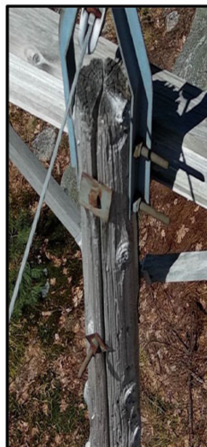
Line M127 Structure 187 Major splitting, rusting hardware
